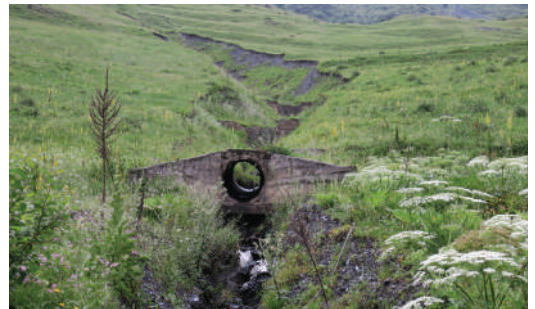
Figure 34: Gully erosion, view from the village, July 2016
