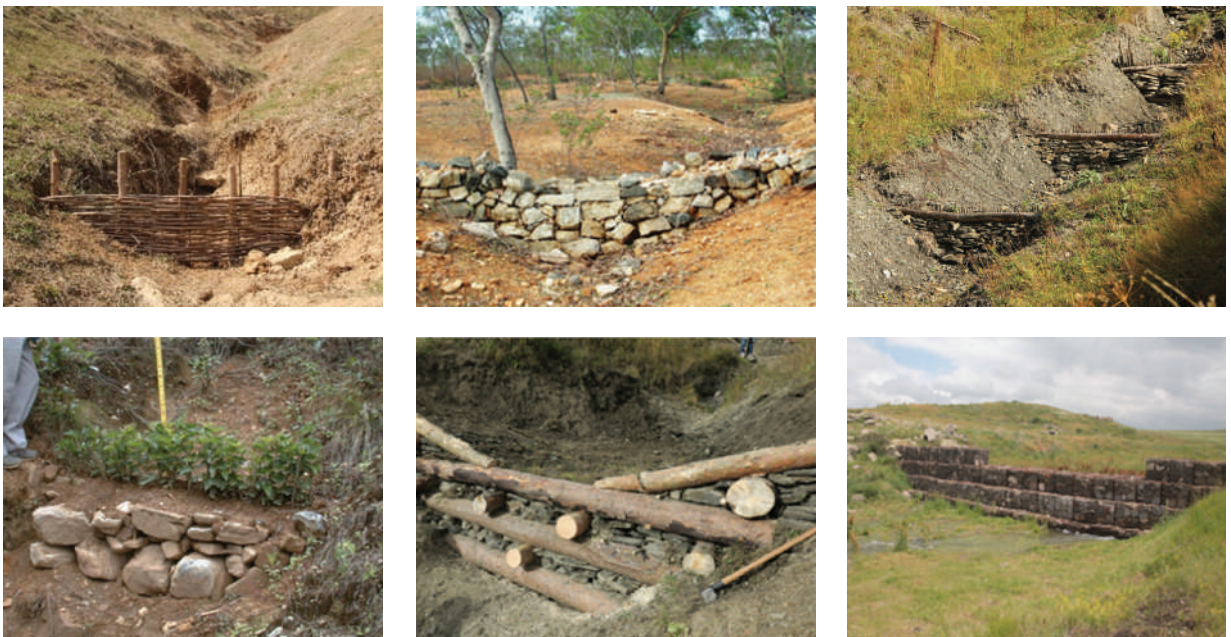
Figure 22: Gully plugs constructed with different materials
